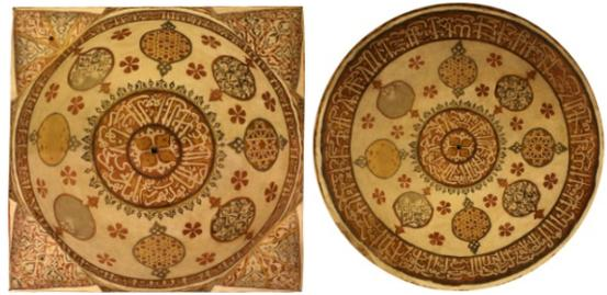
**Figure 9 :** Simultaneous use of laser and images to produce orthophotos of a cupola (orthogonal and azimuth projection).
